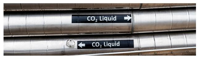
Liquefied carbon dioxide (LCO $_2$ ) is a fluid obtained by cooling the CO $_2$  between  $-35\,^{\circ}$ C and  $-15\,^{\circ}$ C reducing its volume approximately by 600 times. This operation is extremely important to enhance the storage and transportation efficiency.
